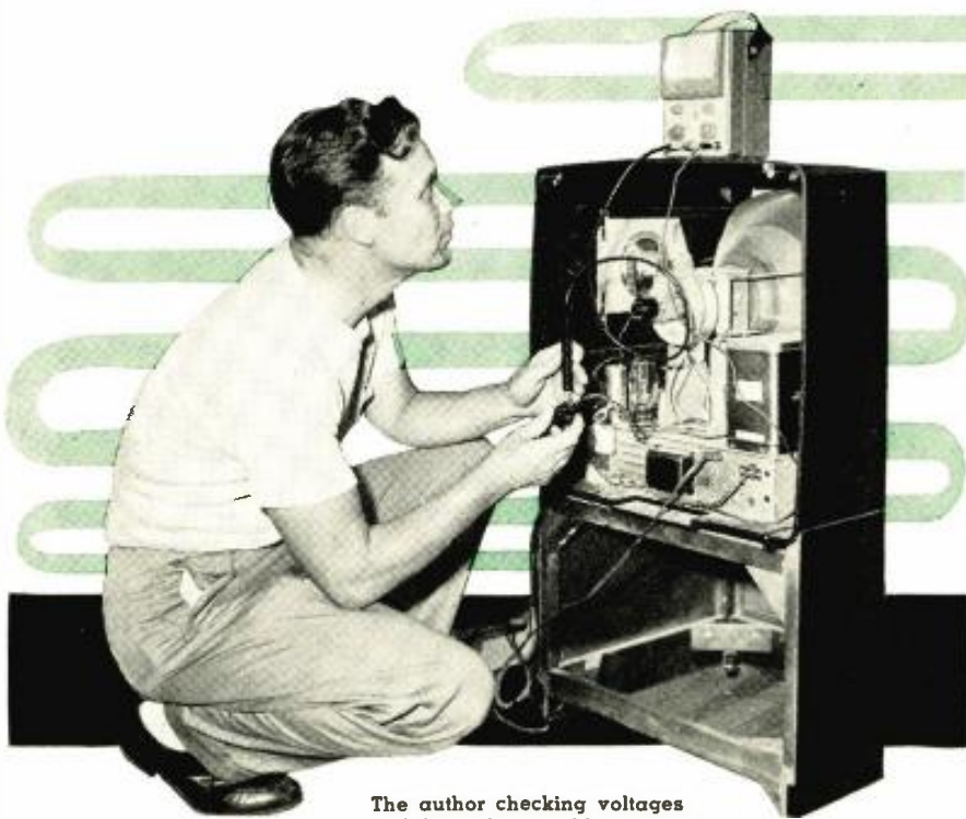
The author checking voltages with his indispensable v.t.v.m.
