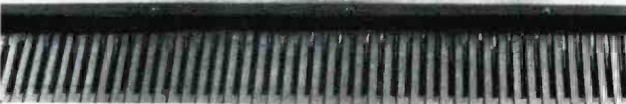
Fig. 30. Rear view of the filterboard taken from the front of the organ console.
